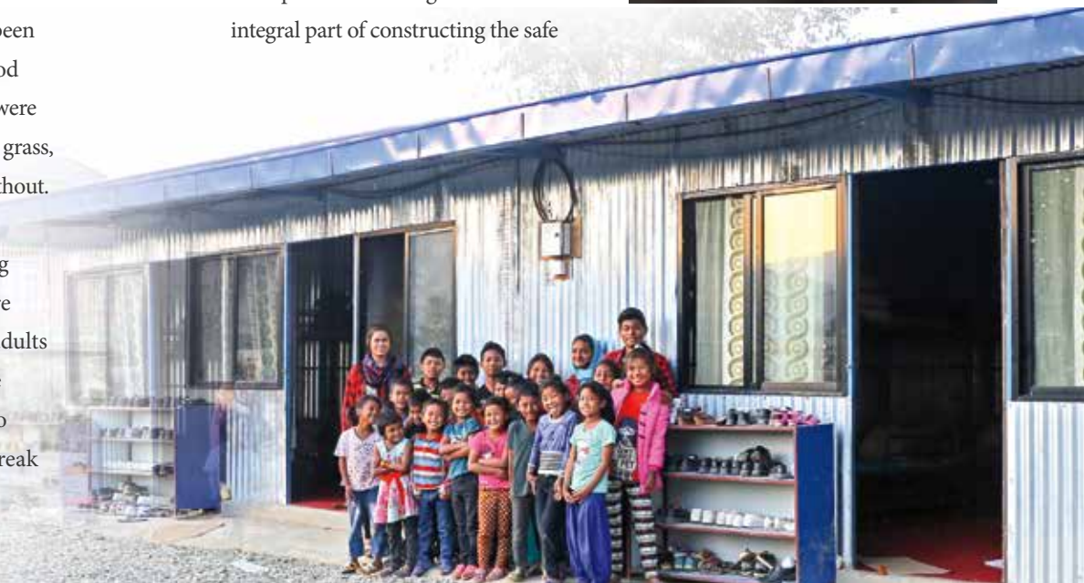
Operation Blessing builds a home for Ganga and other children in need of safe shelter.
